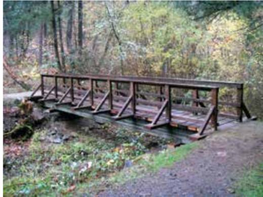
A new bridge now crosses Jackson Creek on the Sarah Zigler Trail. After over 15 years of use, the original foot bridge was determined to be suffering from long term exposure to the weather, dry rot and age. The bridge replacement, which took place last fall, was a joint project between the City of Jacksonville and The Jacksonville Woodlands Association.
