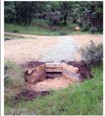
*This wooden cut-off collar will help collect running water, and force it through the French drain (gravel-filled ditch) on its journey down the drainage..*
